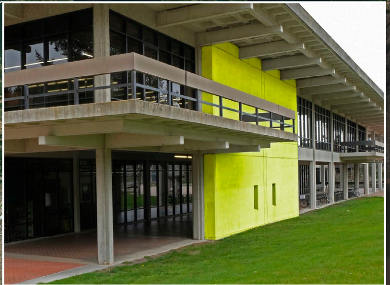
This is just one of the many seismic mitigation projects completed across the Evergreen State College campus. In this photo you can see the shear wall (highlighted in yellow) that was installed to reduce lateral movement of the building during seismic events.
